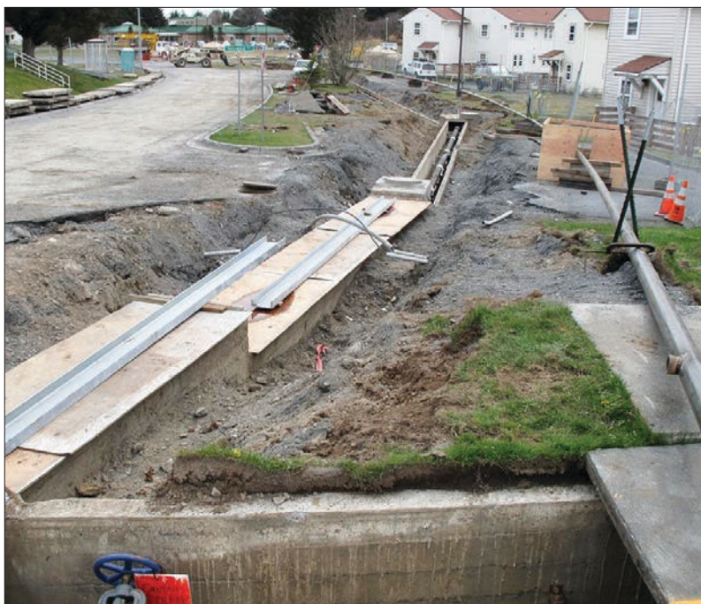
Steam lines are repaired at Coast Guard Base Kodiak in Alaska. Civil Engineering Unit Juneau's Environmental Management Branch provides environmental restoration and compliance services to support Coast Guard operations throughout the state. This includes managing environmental concerns, ensuring compliance with regulations, and addressing issues related to energy conservation and hazardous materials. Coast Guard photo by Brian Goettler
