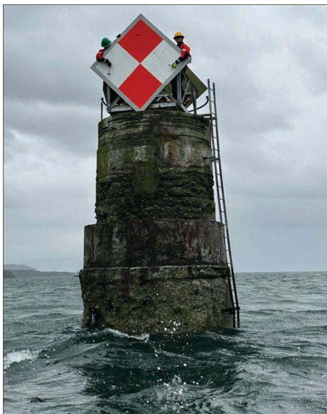
CGC Elderberry crewmembers renew a day board. Coast Guard personnel assigned to the 65-foot inland buoy tender service 285 of Southeast Alaska's 855 aids to navigation. Coast Guard photo
